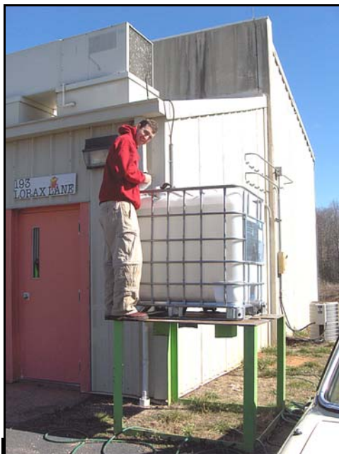
Tim at work on the rainwater catchment system at Piedmont Industrial
